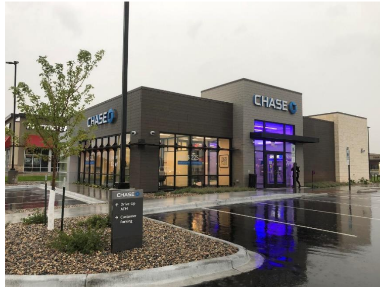
Data Line Installations
