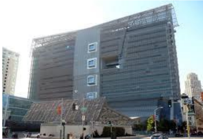
(Government) Social Security Office Software Installation, Fiber Optic Installation for entire building, Installed new Network system
