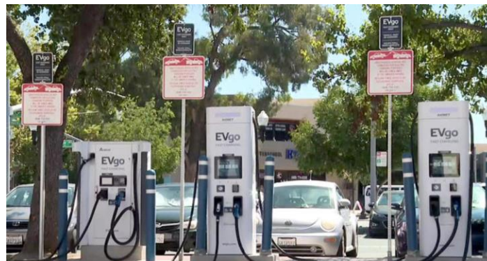
Installation of New Electric Vehicle Station
